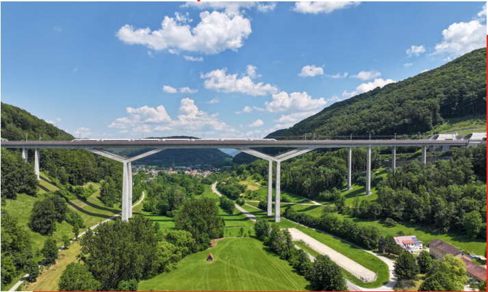
Filstal Bridge at Mühlhausen
